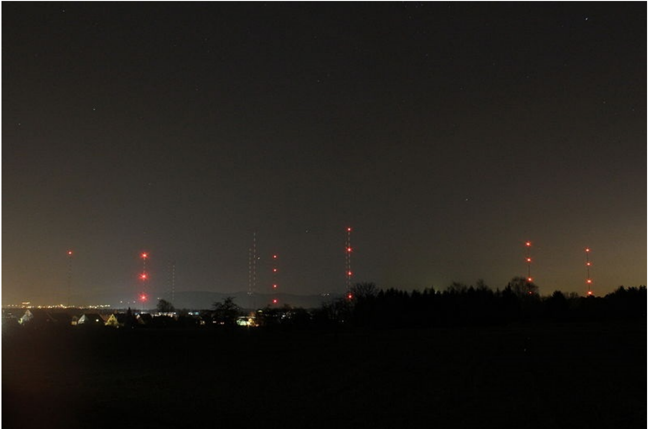
Figure 1: The low frequency T-aerial antennas of the continuously operated DCF77 signal in Mainflingen at night.
